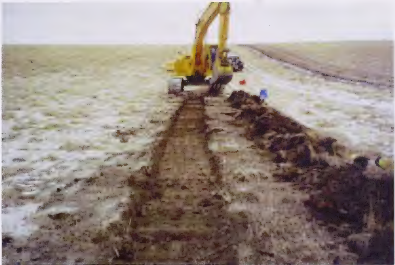
Photo 29 Trench line stripping in frozen ground conditions
